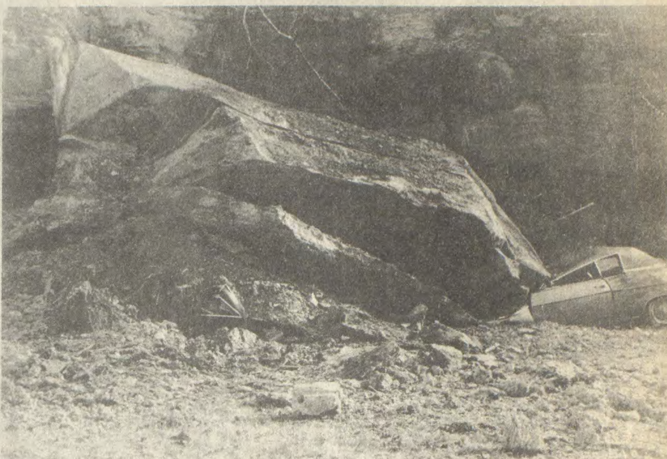
WHEN THE ED CAMPBELL FAMILY AWOKE Monday morning, they discovered that they had narrowly escaped the fate of the two cars lying under this massive rockfall. Their trailer is located just a few feet from the fall on the Mountain Parkway near State Road Fork.
