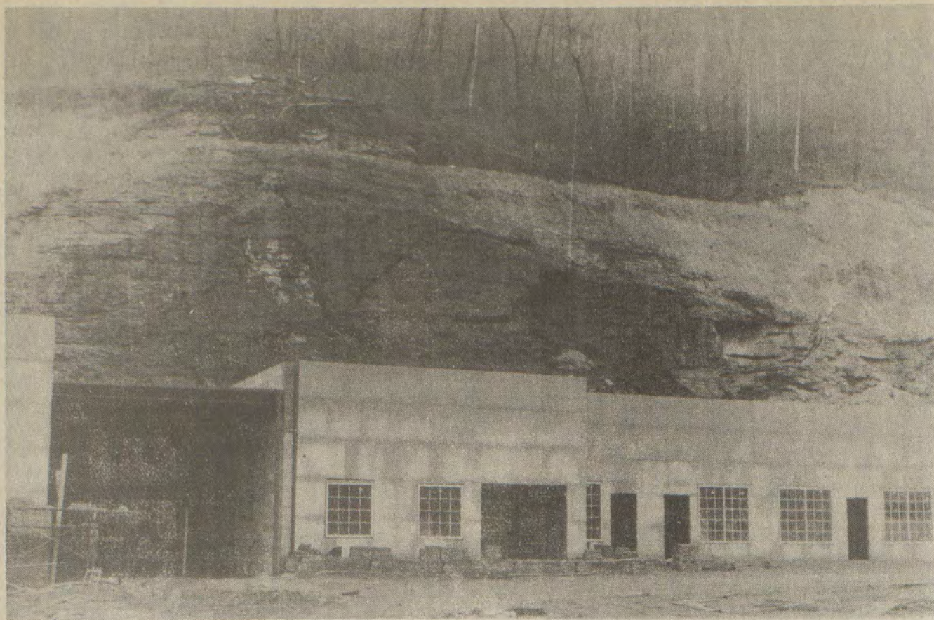
A HORIZONTAL FISSURE was noticeable this week on the highwall rising behind a partly-finished building on the site of the Prestonsburg Village Shopping Center. Concern for the safety of the cliffs bordering the site has prompted city code enforcement officials to suspend construction there.
