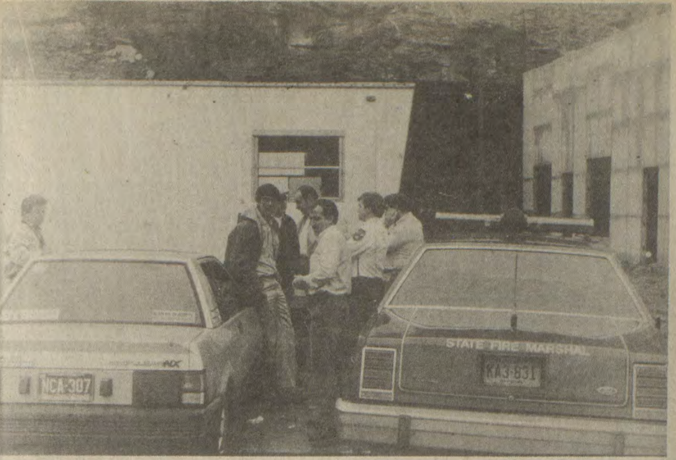
STATE AND CITY officials conferred with developers Tuesday on the site of the Prestonsburg Village shopping center, construction of which has been halted pending further investigation of the hazards presented by the sheer cliff faces surrounding the project. A second engineer's report on the problem is expected this week.
