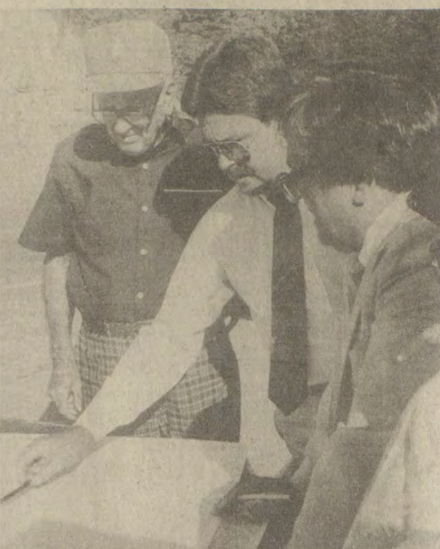
APPROACHES TO THE NEW CLIFF BRIDGE continue to be of concern to residents of the Abbott Creek and Cliff areas. Meeting Tuesday at the bridge site, Delmas Saunders, State Representative Greg Stumbo, and Kirby Ison, Jr., chief highway engineer, studied a map of the trouble spot. Senator David LeMaster was present for the meeting as were several others.
