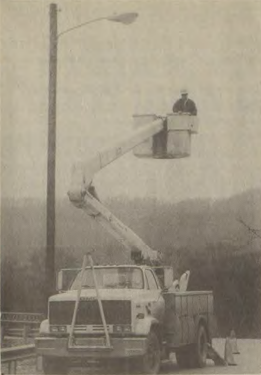
LIGHTS WERE INSTALLED this week at entrances to the new Cliff access road. Their installation was approved at a recent meeting of the Prestonsburg City Council to aid motorists utilizing the new route.
