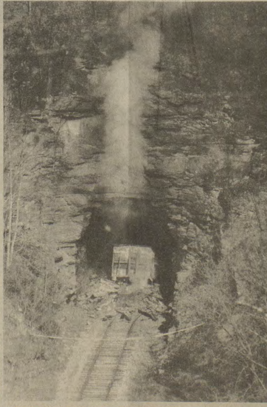
TIMBERS IN THIS RAILROAD TUNNEL near Hi Hat are expected to continue burning for perhaps three weeks. The blaze apparently began between 9 and 9:30 Thursday night, with "an explosion, but not like dynamite, like a fire roaring," according to Ronnie Meade, whose home is near the tunnel. Meade's son, James, first noticed the flames shooting from the mouth of the tunnel as high as 200 feet into the air shortly after 9 o'clock. Although Sheriff's Deputy Harold Johnson said he suspected arson, officials of the C&O Railroad and Kentucky State Police said Monday their investigations are incomplete.
