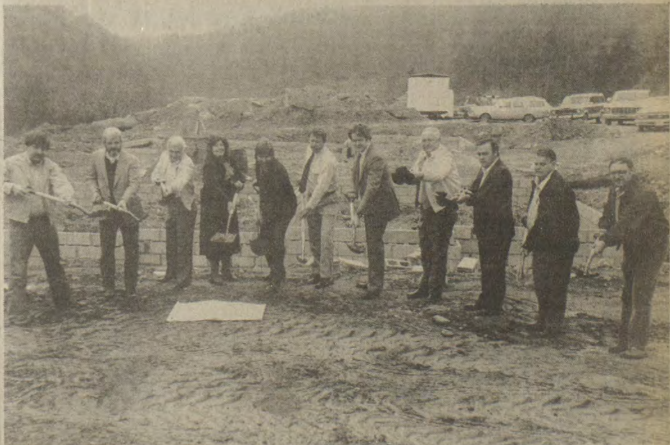
Although foundation work is already well under way, ground was officially broken Friday for the county's newest public housing development on Ivy Creek at Ivel. A project of the Floyd County Housing Authority, the complex will provide 41 two, three and four-bedroom townhouse-type dwellings at a total cost of near $2.5 million. Most of the funding is being provided by the federal Department of Housing and Urban Development (HUD) with additional grants from the Appalachian Regional Commission and the Kentucky Housing Corporation's Land Grant Program. On hand for the groundbreaking were, from left: Paul Hunt Thompson, Floyd County Housing Authority board member; Morris Hylton, board member; Wendell Stratton, Ivel civic leader; Julia May, executive director of the Floyd County Housing Authority; Bill Richardson, project architect, of Whitesburg; Ron Reynolds, C.B. & S. Construction Co., Lexington; Congressman Chris Perkins; Floyd County Judge-Executive John M. Stumbo; Burl Shepherd, chairman of the Floyd County Housing Authority; Ray "Shag" Campbell, Floyd county school board member, and Eddie Patton, housing board member.
