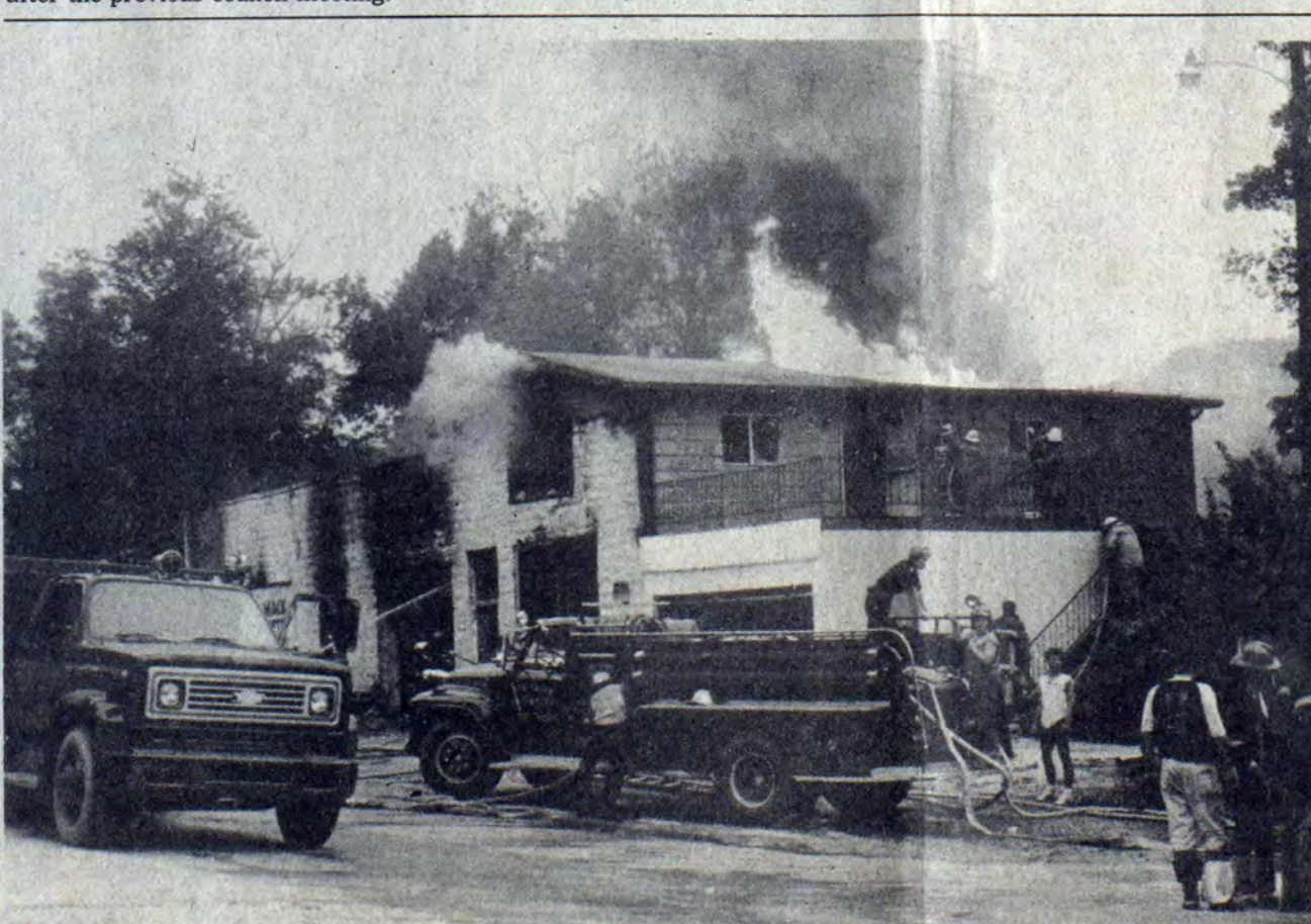
SCENE OF FIRE which last Tuesday evening destroyed the Mountain Truck Parts building at Allen. Area firefighters joined in a futile battle against the blaze which is believed to have originated from the nearby burning of garbage. The structure, which also included the upstairs residence of George Allen, was the scene, nearly three years ago of a mass slaying in which five men were killed and three wounded by then 72-year-old William Okie Bevins, of Printer.
