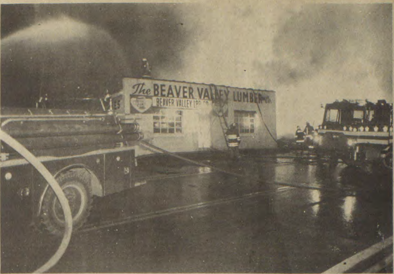
FRIDAY MORNING'S FIRE at Martin which burned a large part of the Beaver Valley Lumber Company, also knocked out power lines and phone service to the town for several hours. Fire departments from all parts of the county combined to restrict the flames from spreading to nearby homes and businesses.
