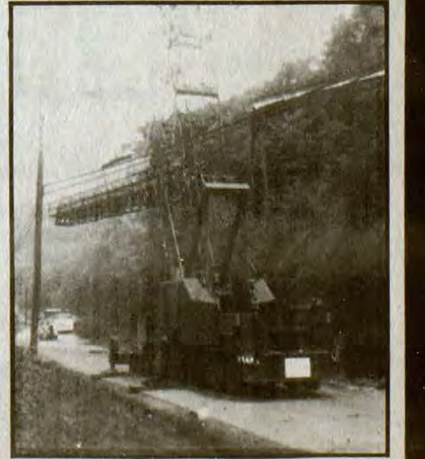
CONVEYOR INSTALLATION AT KENTUCKY CARBON AT PHELPS, KY.
