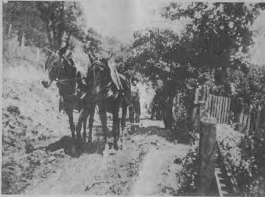
This old picture of Ellis Conley was taken back in 1936 when the "new" road up Salt Lick Creek, near Hueysville, was being built. Conley is pictured with his mule team, consisting of Barney and Gyp, guiding a slip scraper along the route during construction. The photo was made in the area of the "Yankee" Jack Allen place. Figure barely visible at right is believed to be Fair Hicks, leader of the work. Photo was submitted by Ellis's son, John B. Conley, now of Chillicothe, Ohio.
