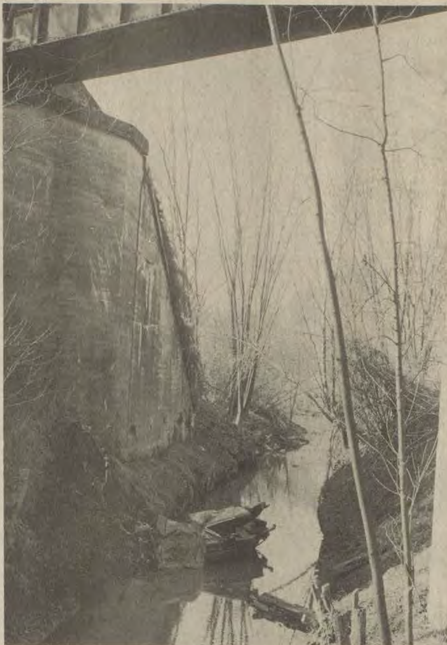
WRECKAGE OF AUTO struck by train at Lancer last Friday night rests in shallow water beneath the railroad trestle from which it toppled. Patty Adkins, 17, of Grethel, and Carolyn Hall, 12, of Galveston, were freed from the wreckage, virtually unharmed.
