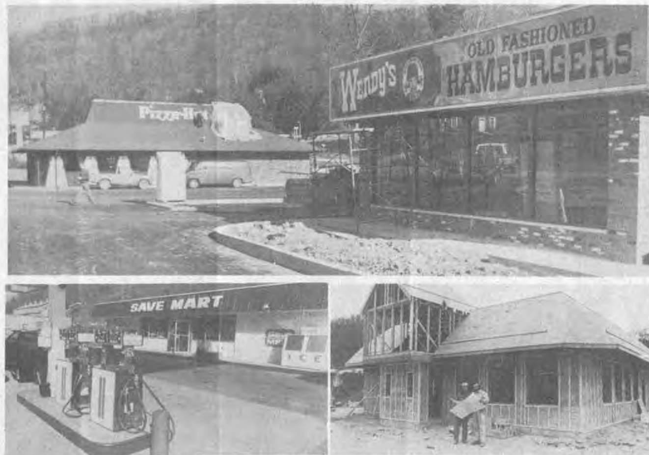
Wendy's and Pizza Hut pictured in top photo at mouth of May's Branch location. New Save-Mart store is shown at upper left, and David contractor Mike VanHoose (at right) is shown with a fellow workman in front of the new Captain D's seafood restaurant.
