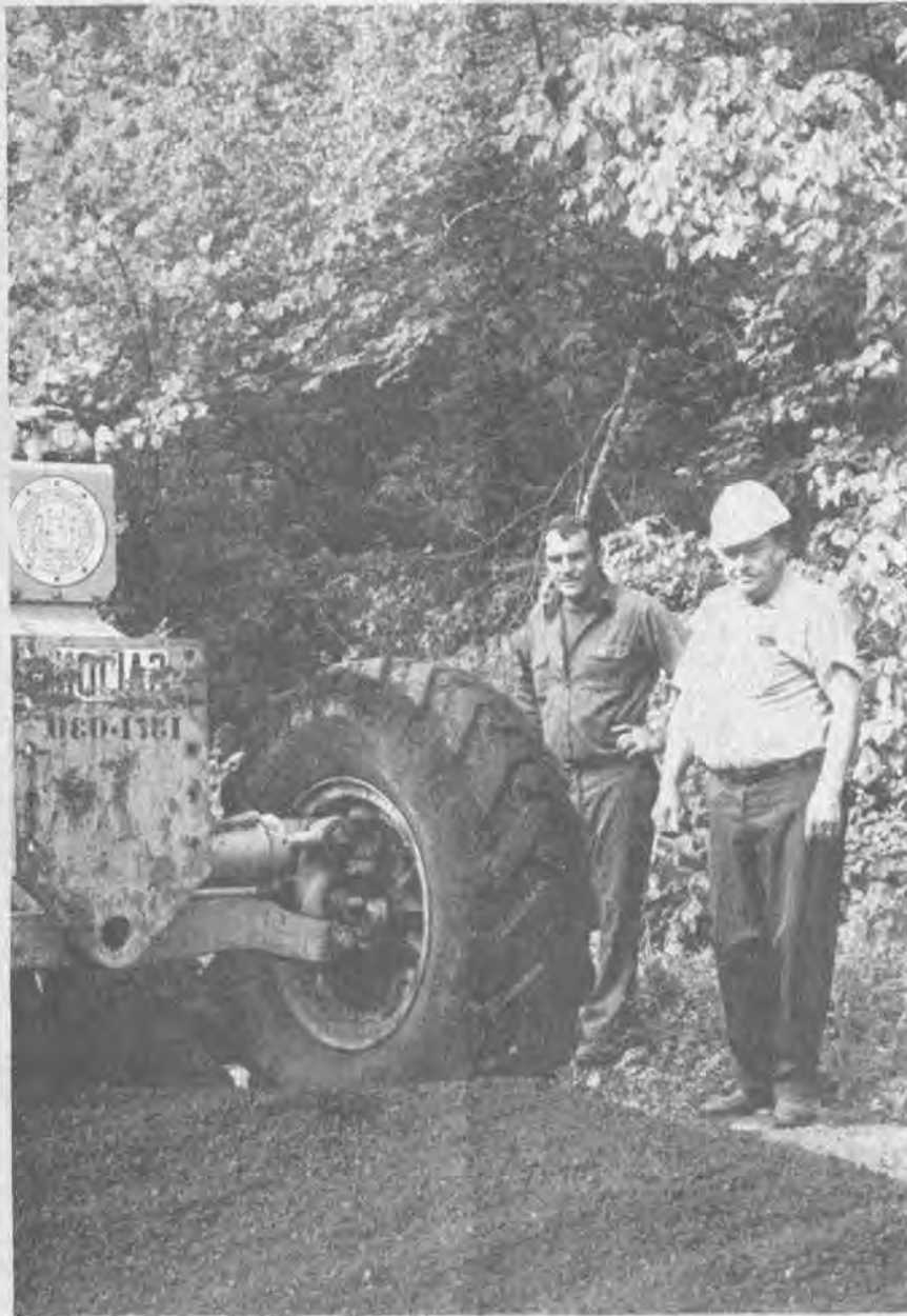
AS THE RESULT OF AN AGREEMENT said to be the first of its kind in this county, a coal operator and state highways authorities jointly undertook repair of the Turkey Creek road last week.
