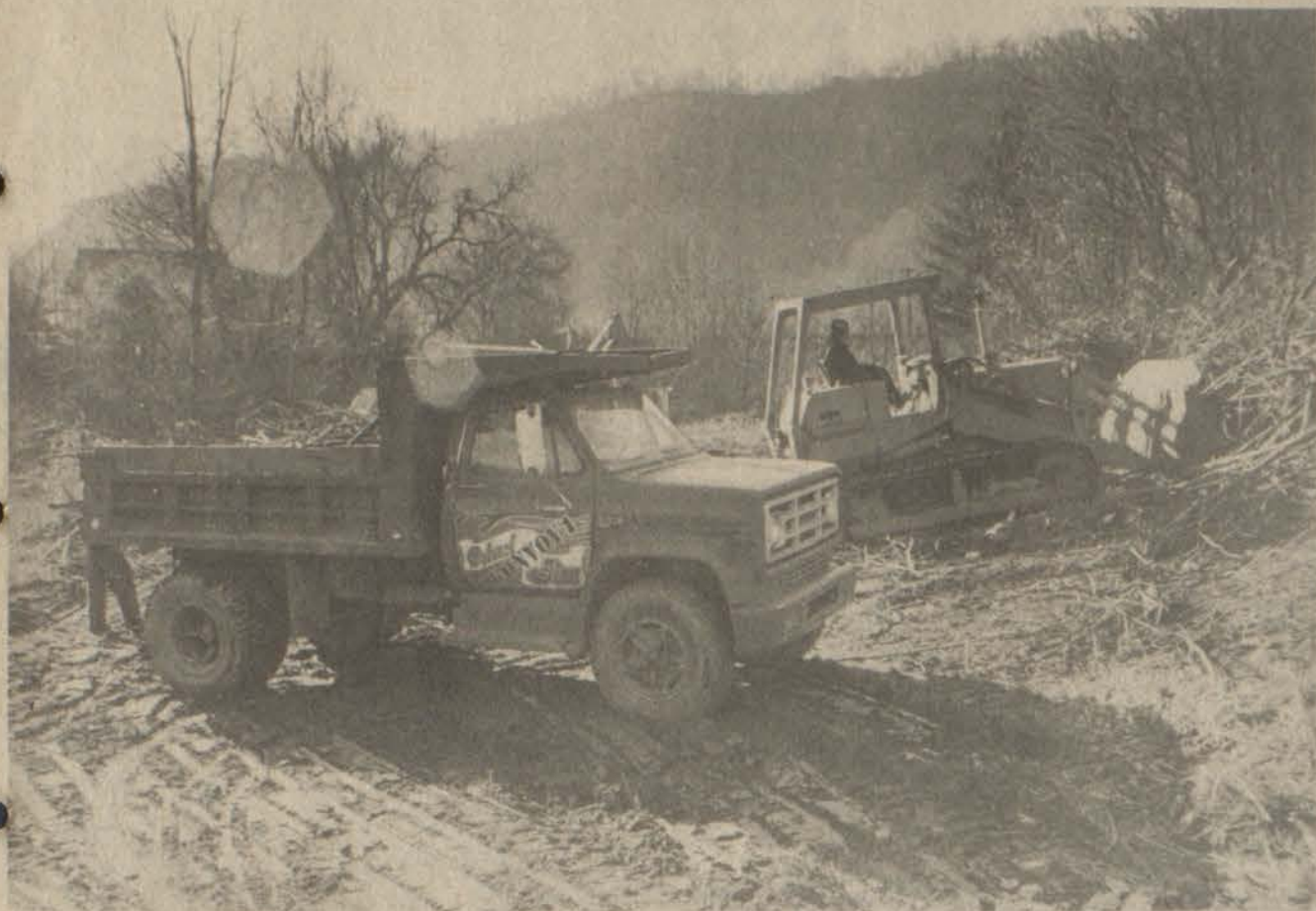
CLEARING AND SNAGGING operations began recently on Beaver Creek at Martin. The work, which is being done under contract with the Army Corps of Engineers, is expected to be completed next month.
