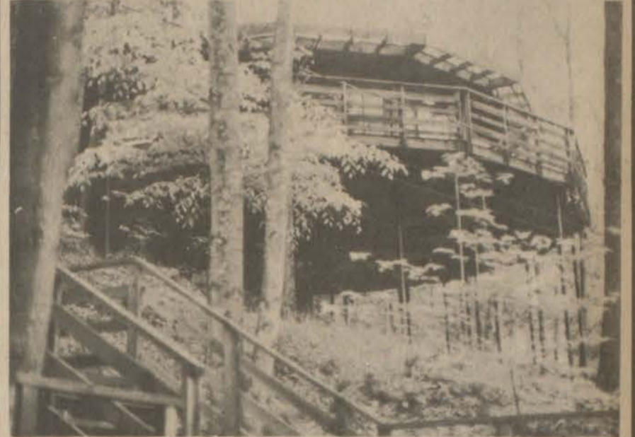
Round house (pictured) located on private property overlooking Dewey Lake in Jenny Wiley State Park. This chalet home has two completely furnished bedrooms, loft area furnished, living and dining room all completely furnished. All appliances and custom-made draperies. Shown by appointment only.
