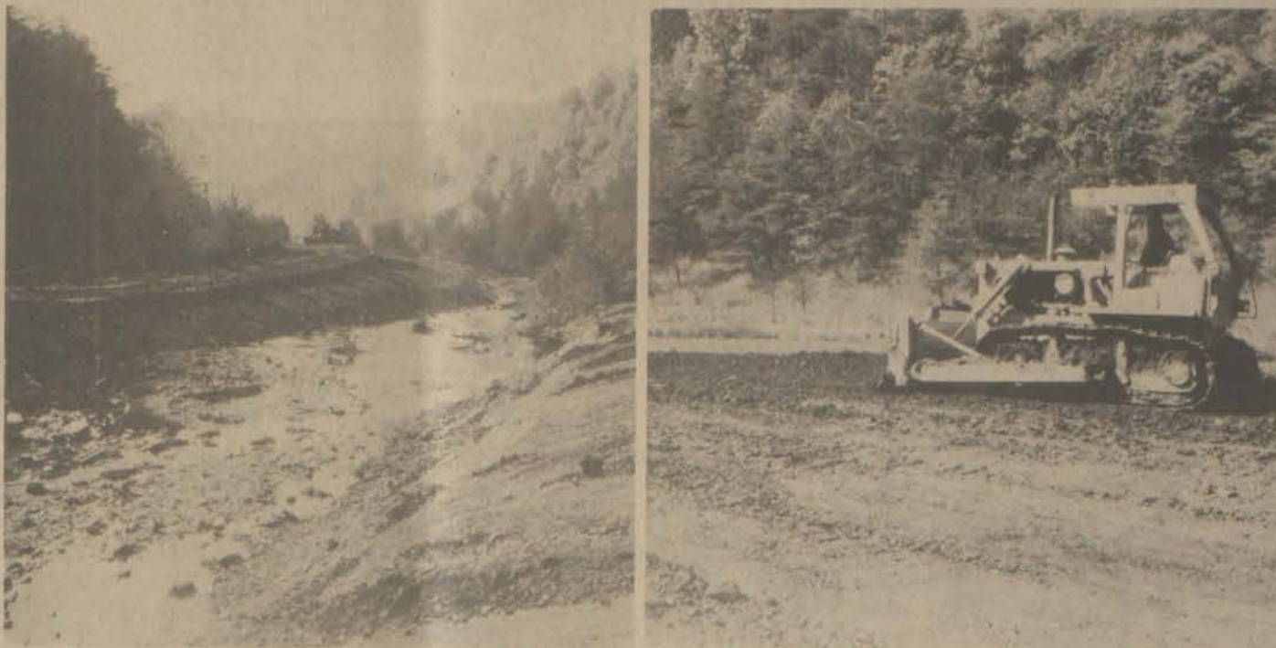
Before (left) and after reclamation work now under way on David Community Development Corporation land. The work is being done under the Rural Abandoned Mine Program, which is administered by the U. S. Soil Conservation Service.
