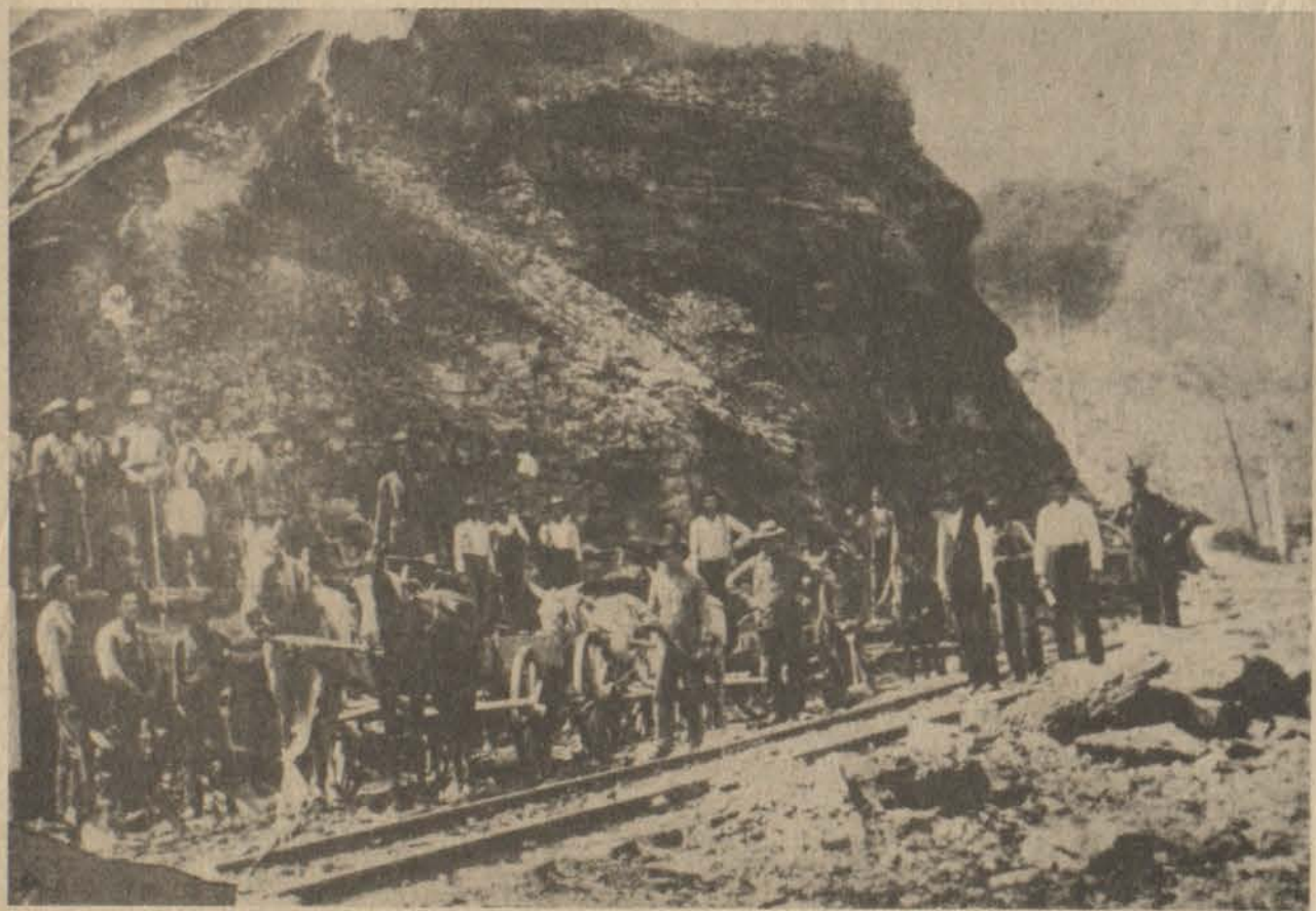
Railroad construction near Prestonsburg. (Courtesy Alice Lloyd Photographic Archives, Henry Scalf Collection.)
