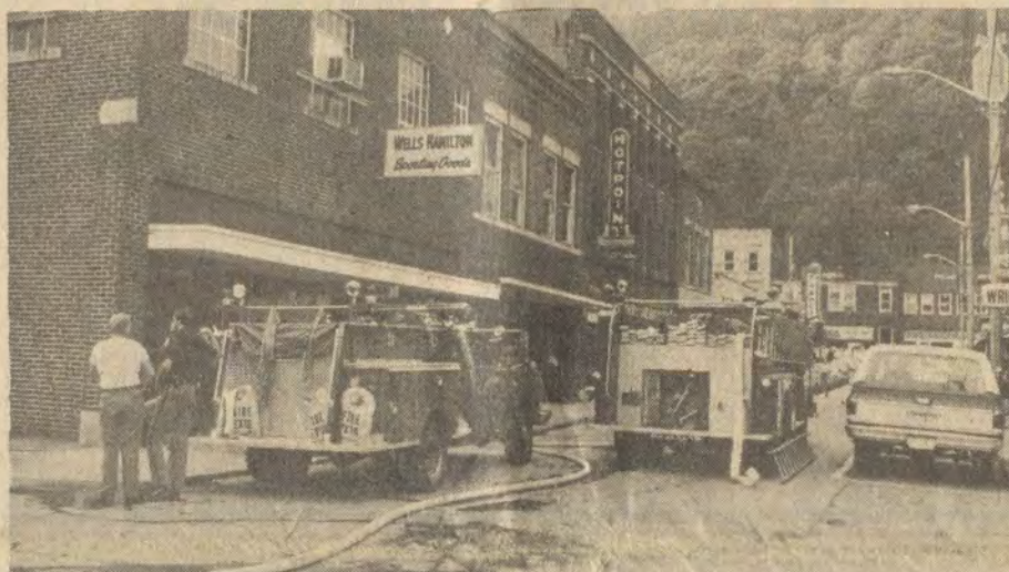
Although little damage resulted when an electric line in a wall of Wells-Hamilton Sporting Goods overheated late Tuesday morning, the potential for a serious blaze downtown caused the Prestonsburg Fire Department to block the Court Street section to traffic for about two hours.
