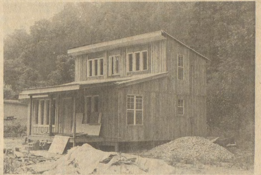
Passive solar energy use and air-dried lumber are features of this experimental house under construction at David. The builders, Appalachian Housing Industries, hope to complete construction this month.
