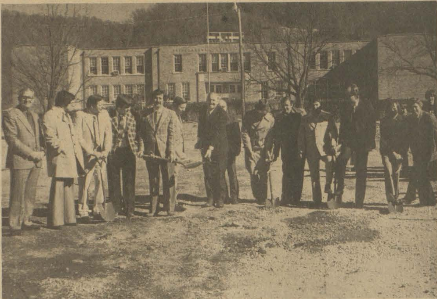
Ground was broken Friday at the North Lake Drive site here of the $690,000 Prestonsburg Municipal Building. Special guests at the ceremony were Congressman Carl D. Perkins and Charles Mason, Kentucky representative of the Economic Development Administration (EDA). Mason called the scheduled construction "one of the most significant projects currently being funded by EDA in Kentucky," and praised Congressman Perkins for his part in procuring the federal funds. Pictured from left to right at the groundbreaking are Tom O. McGuire, project contractor; Randy Burchett, representative of Marvin Crider and Associates, architect; Ronald Hager, Donald Nunnery and Paul Phillip Hughes, city councilmen; Prestonsburg Mayor Harold Cooley, Congressman Perkins, City Manager Curtis Clark, Mr. Mason, and Edgille "Shag" Branham, George Cecil Brown, Dr. Larry Leslie, Cloyd Johnson and Hansel Cooley, city councilmen. The new facility will house all offices of Prestonsburg city government, including the police and fire stations.
