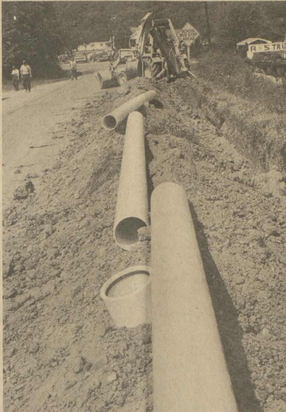
Excavation work in progress last week on new water service.
