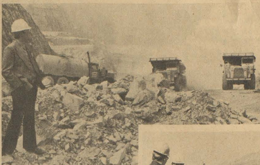
(ABOVE) Moving mountains isn't something you do overnight, but the Kentucky Department of Transportation's district highway office at Pikeville has made impressive headway in slicing through 13.5 million cubic yards of rock in Pike County. The huge cut is the heart of a multiple agency, model city project, which will provide more building space in Pikeville. It will allow removal of a railroad line from the city, rechanneling of the Levisa Fork of Big Sandy River away from the city, and building a new four-lane section of U.S. 23.
