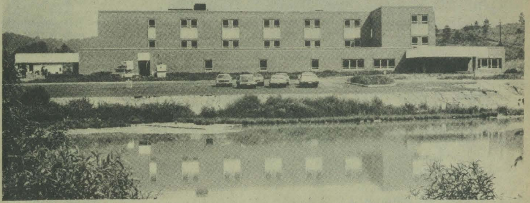
HOSPITAL NEARS COMPLETION.—The new Louisa Community Hospital, developed by Humana, Inc., the Louisville-based hospital company, is nearing completion on a 10.8 acre site on Highway 644, about two miles south of the Louisa business district and across the highway from a site for a new high school.
