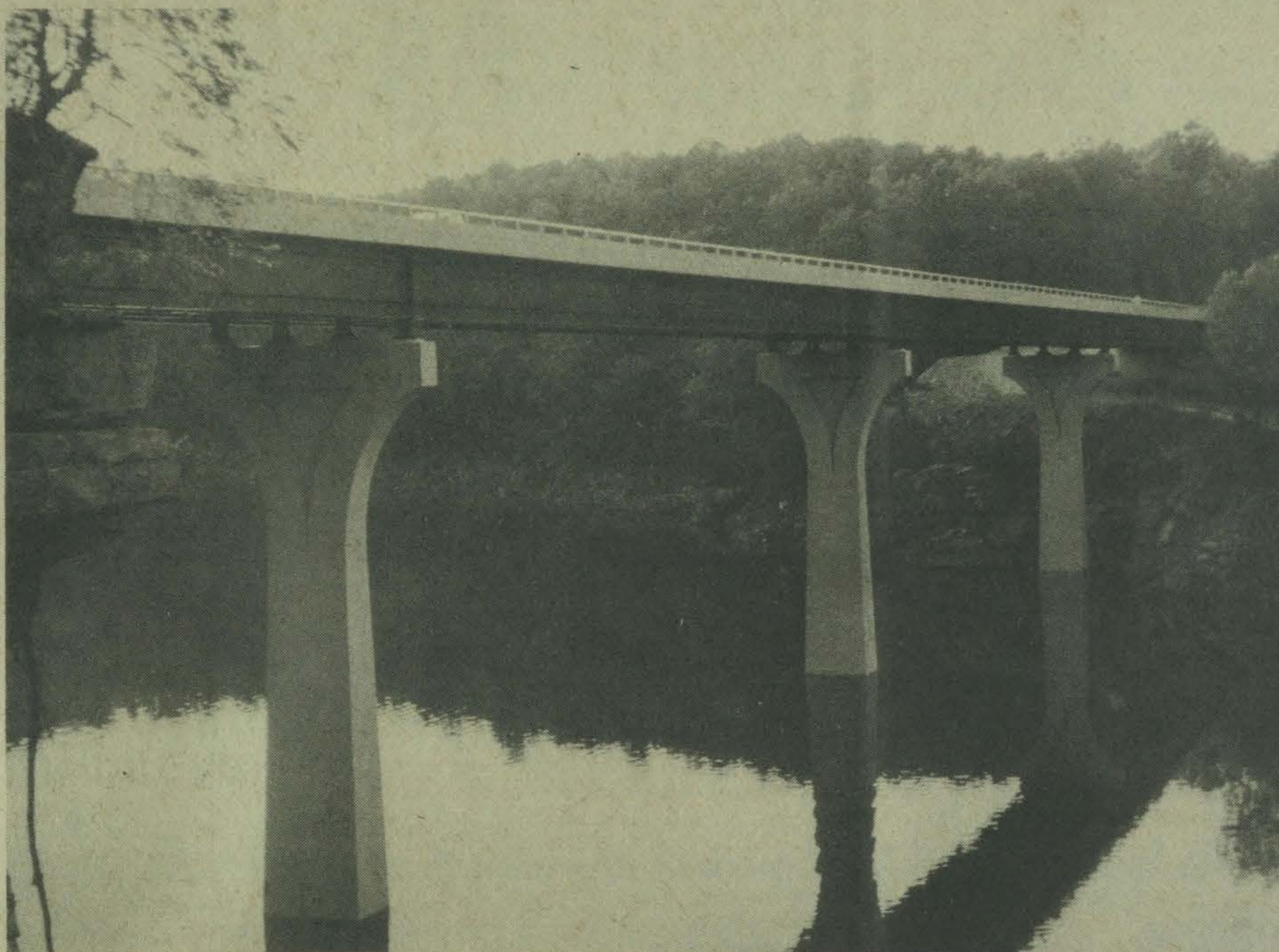
This new bridge, which opened recently near Corbin, was built by Prestonsburg contractor Joe A. Burchett, of Bush & Burchett, Inc., Frankfort, Ky., and was designed by the Nashville District, U. S. Army Corps of Engineers. The $1.1 million span crosses the Laurel River and is near Kentucky's newest lake, Laurel River Lake, which was impounded for hydropower generation and recreation.
