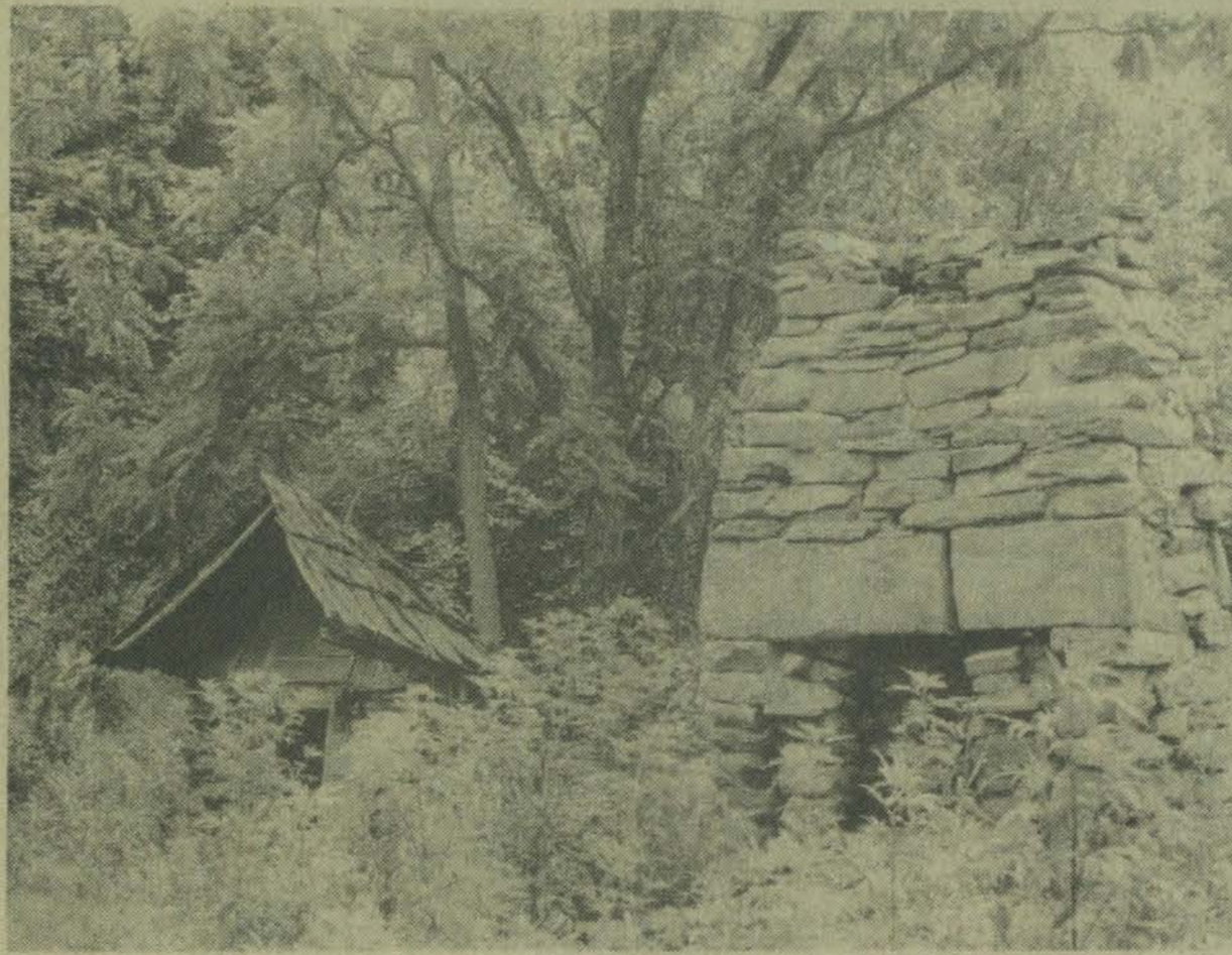
The ruins of this chimney, one of the few remaining signs of a family home on Turkey Creek, can be given life only by a lively imagination which turns to winter scenes and family members before its roaring fire. The small structure at left still houses some of the tools used by the owner, now dead.
