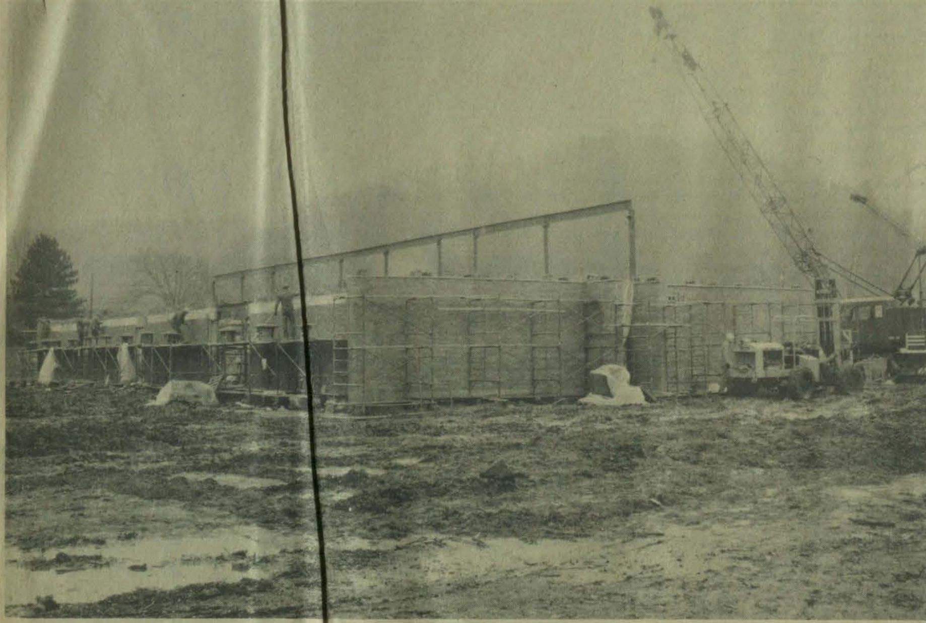
Clinic Structure Under Construction
