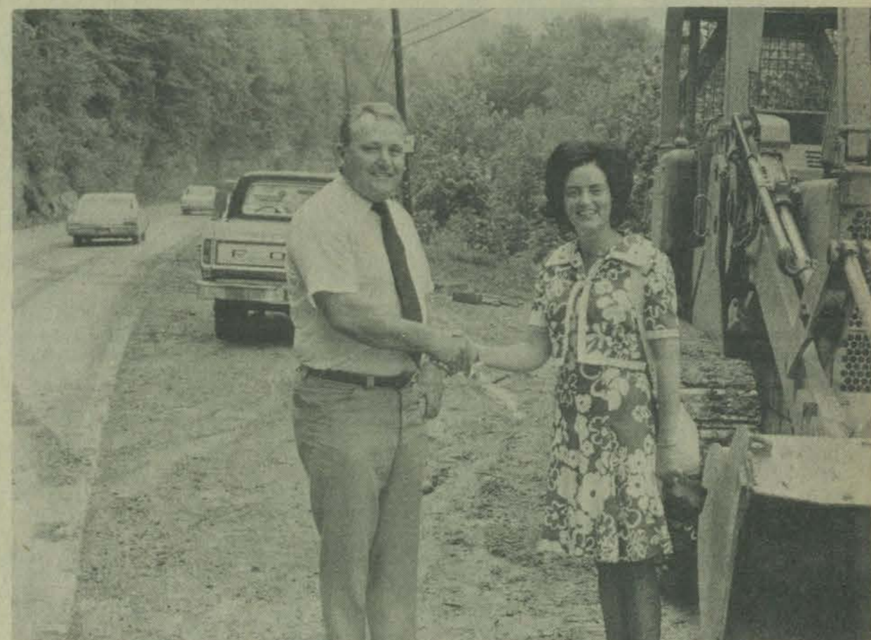
AT SITE OF BRIDGE TO BE BUILT AT EMMA, Marion C. Webb, president of Edwards & Webb Construction Co., contractors on the Emma bridge, congratulates Mrs. Flo Weddington Adams on her successful efforts to win the improvement for her community.
