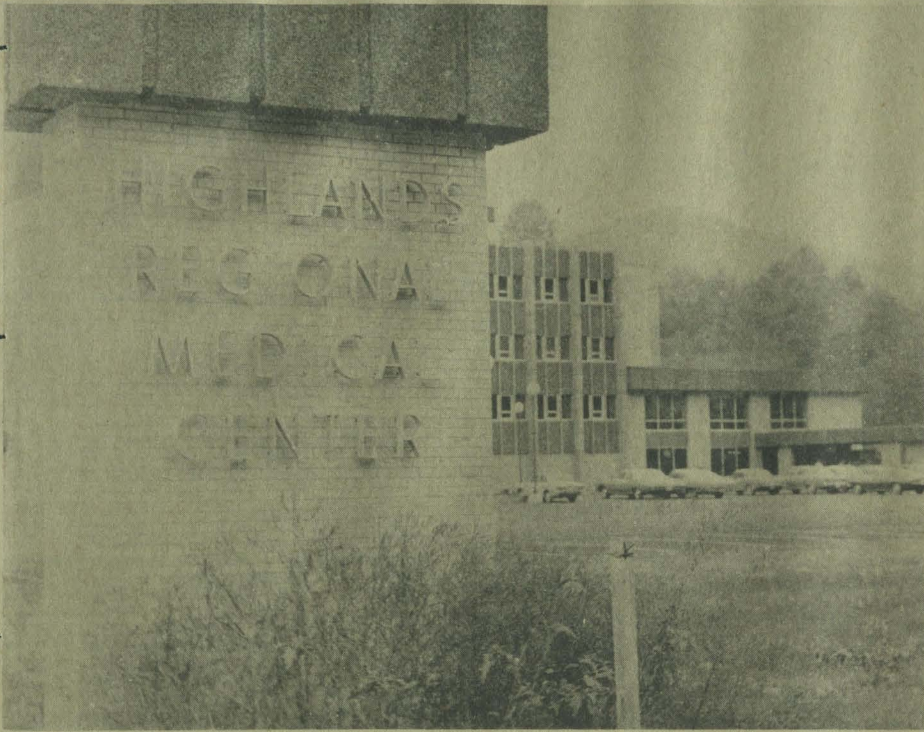
Near-complete Highlands Regional Hospital
