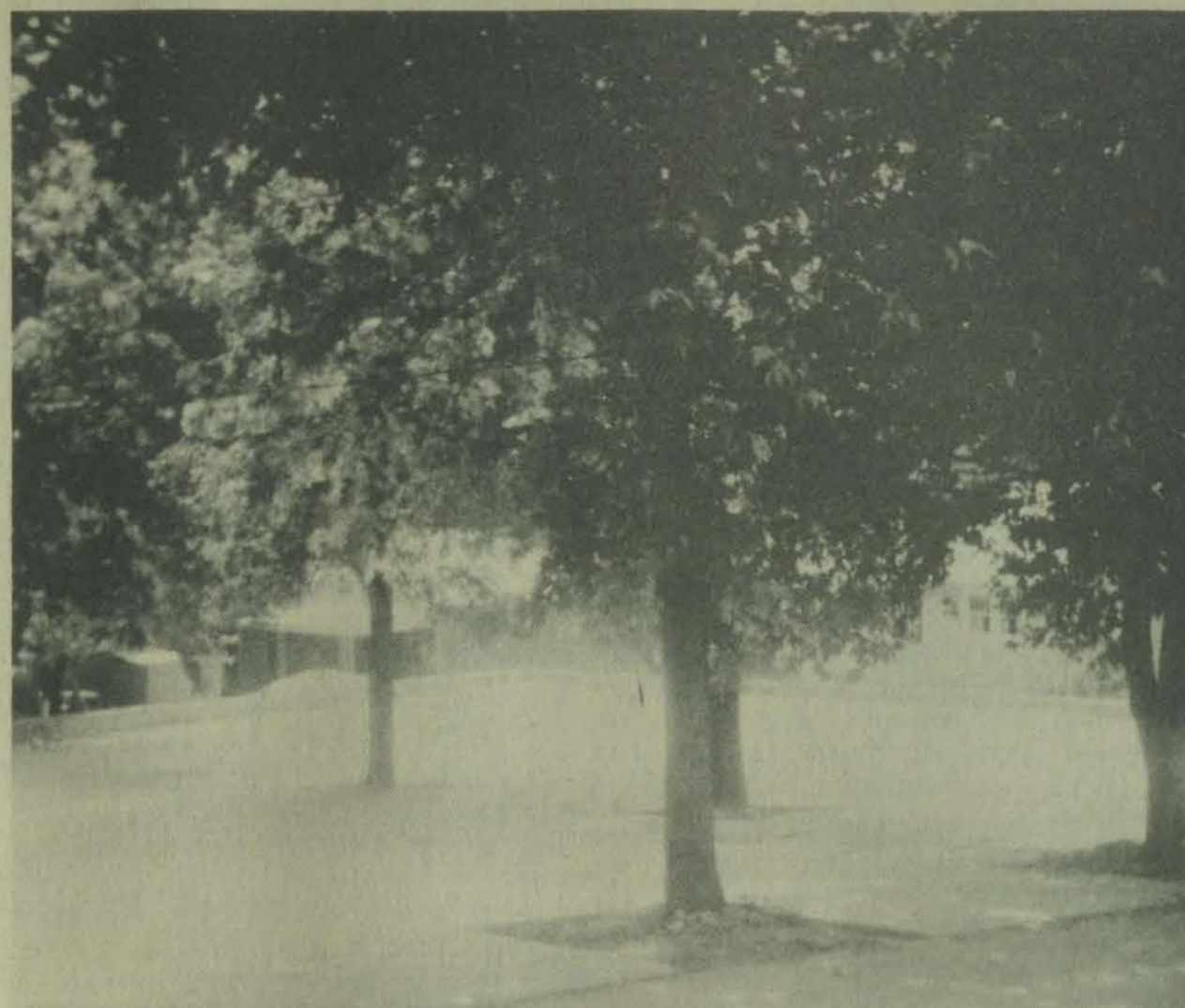
Our Lady of the Way Hospital recently completed construction of a parking lot at the rear of the hospital's clinic in which several of the hospital physician's offices are located. The new parking lot is constructed of concrete and provides parking for more than 20 cars. This has eased the inconveniences and problems which have been experienced by the city of Martin due to a lack of authorized parking in the area immediately surrounding the hospital.
