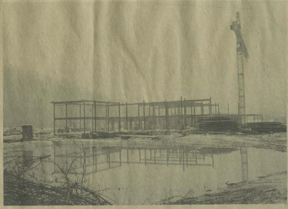
Photo shows steel for the superstructure of the Highlands Hospital under construction near Auxier, but invisible is basement and foundation work which required months to complete. In this underground area will be the dietary department, a cafeteria of 250 seating capacity, general stores, purchasing agent's and engineer's offices, morgue, outpatient offices, refrigeration area and central
