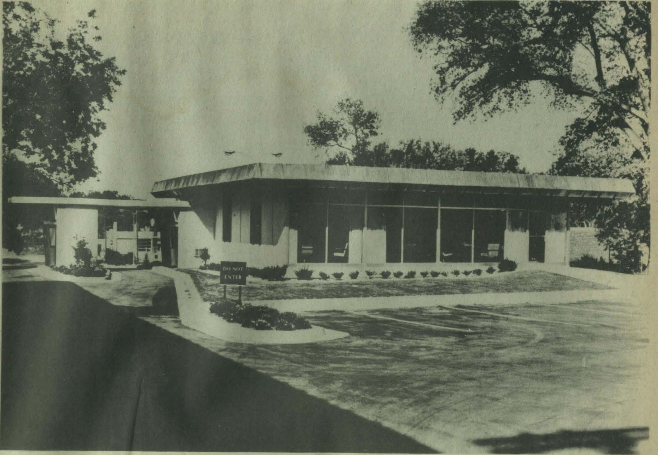
A similar design of what you can see now on our new North Lake Drive location
