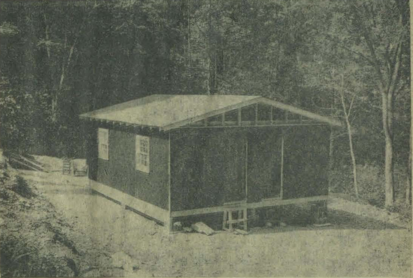
The new home built for Mr. and Mrs. Puckett.
