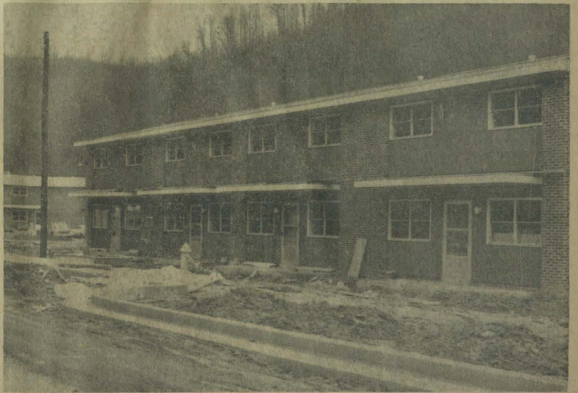
INDIAN HILLS, second public housing complex to be built here, is nearing completion. Photo shows one building of the 42-unit project getting the final touches before occupancy. Indian Hills is located at the mouth of May Branch here, near Green Acres, first housing project developed locally.
