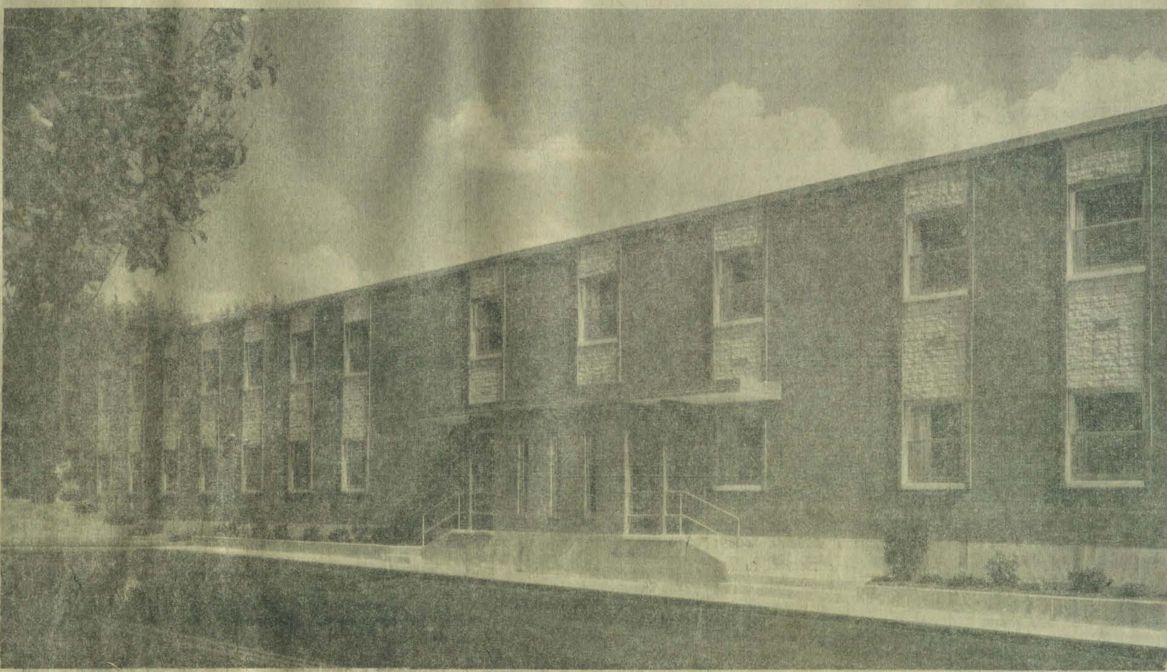
The new 40-bed Our Lady of the Way Hospital at Martin which was dedicated recently. The hospital opened, July 21.
