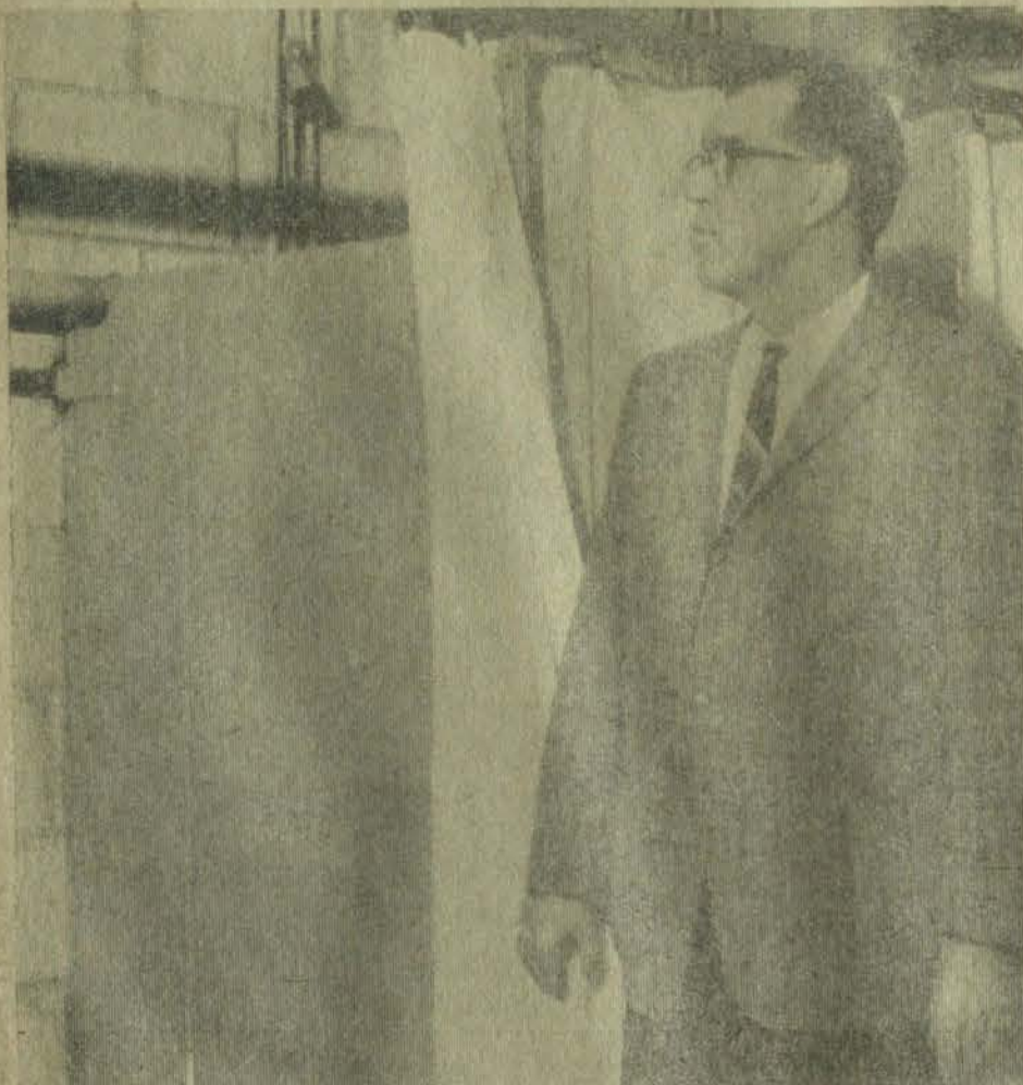
Mayor Archer examines the handwork of work experience and training participants who erected these shower stalls at Archer Park. The showers serve the pool area in the summer and will accommodate athletes using the gymnasium upstairs as well. Materials were salvaged from the county jail, torn down under Prestonsburg urban renewal.
