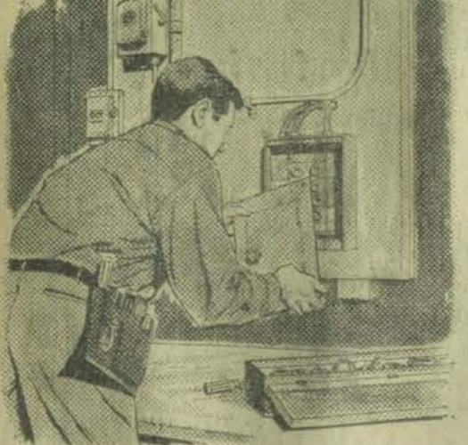
ENTRANCE PANEL (fuse box) must be large enough for your ever-increasing need for more electricity. Inadequate panels can cause trouble.
