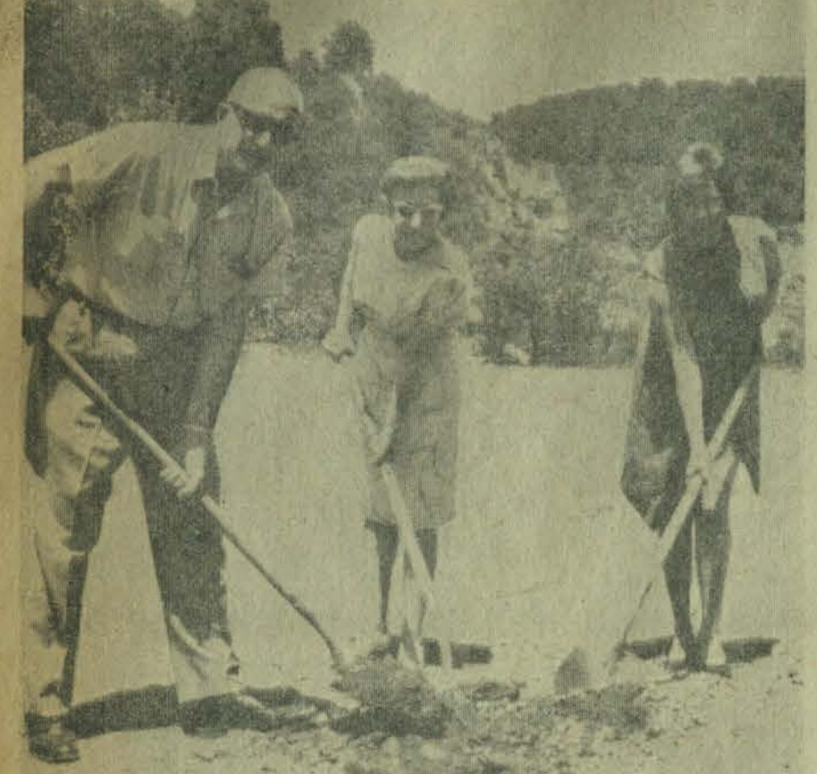
SECOND BUILDING PROJECT BEGUN. Shown breaking ground for the second brick structure to be erected at the new City Park here are members of the Park Board. From left—H. B. Ranier, Mrs. Mary Jane Harkins, Mrs. J. D. Adams.
