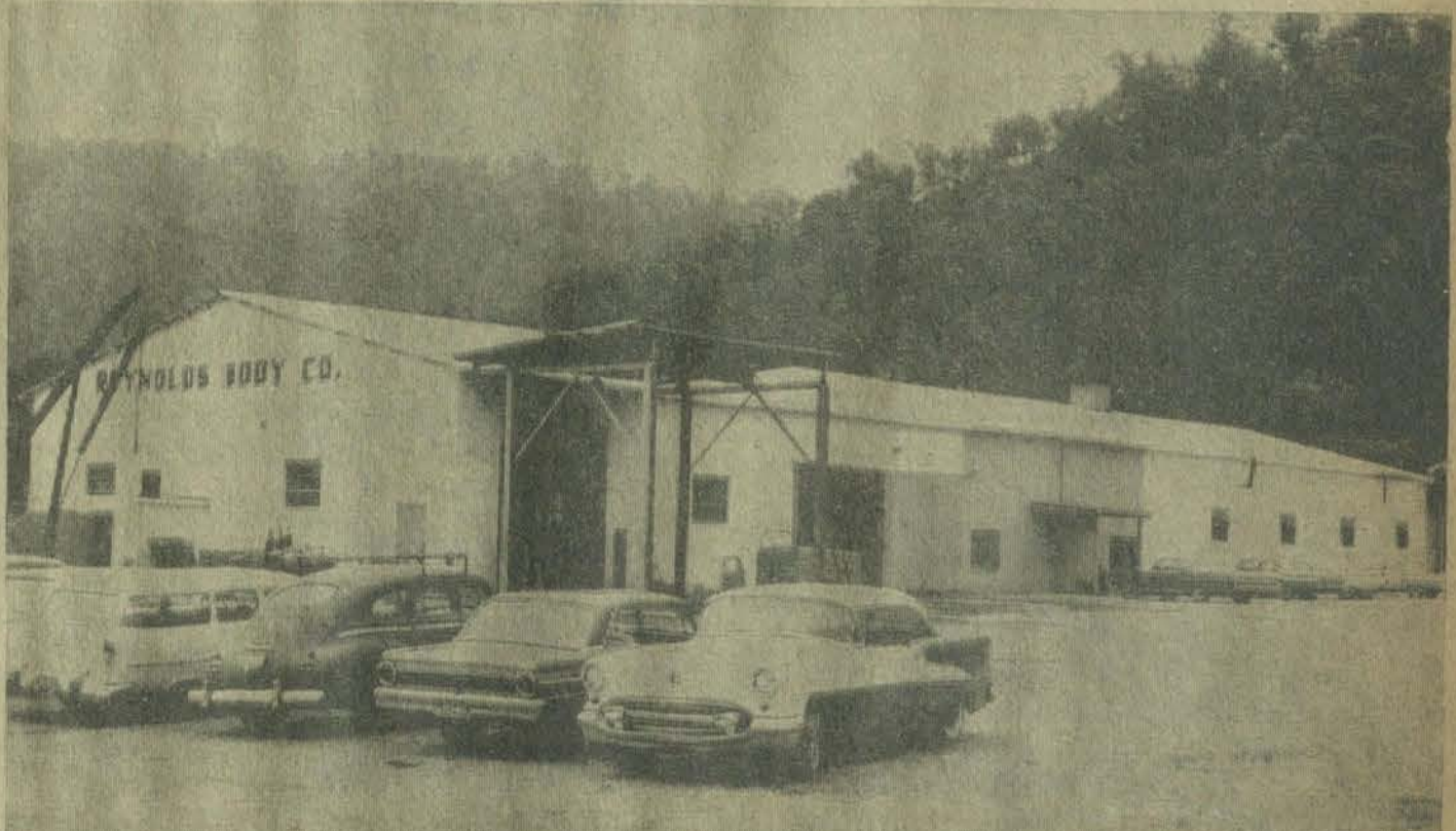
The Reynolds Body Company building, off U. S. 23, near Allen.
