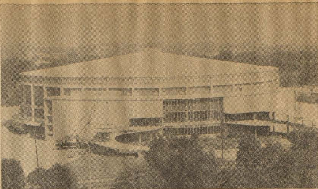
THIS IS WESTERN'S NEW ACADEMIC-ATHLETIC BUILDING. THE CIRCULAR STEEL ROOF IS INSULATED, SUPPORTED BY RADIAL SPANS.
