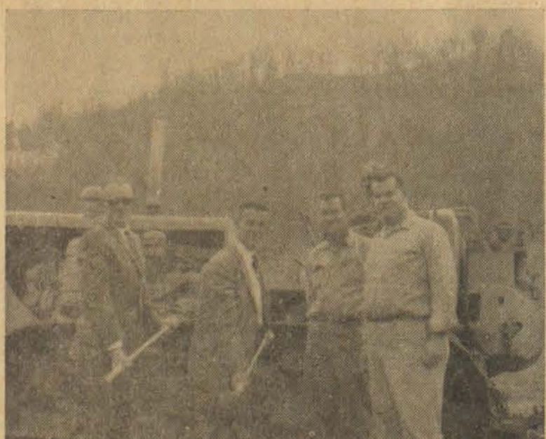
GROUND BREAKING FOR SCHOOL... Ground breaking ceremonies were held March 26 at the site of the projected new Middle Creek elementary school. Shown here, left to right are Lee Shannon, architect, Superintendent Charles F. Clark, Tom O. McGuire, contractor, Bill Clifton, equipment operator, and Clyde VanHoose, contractor.
