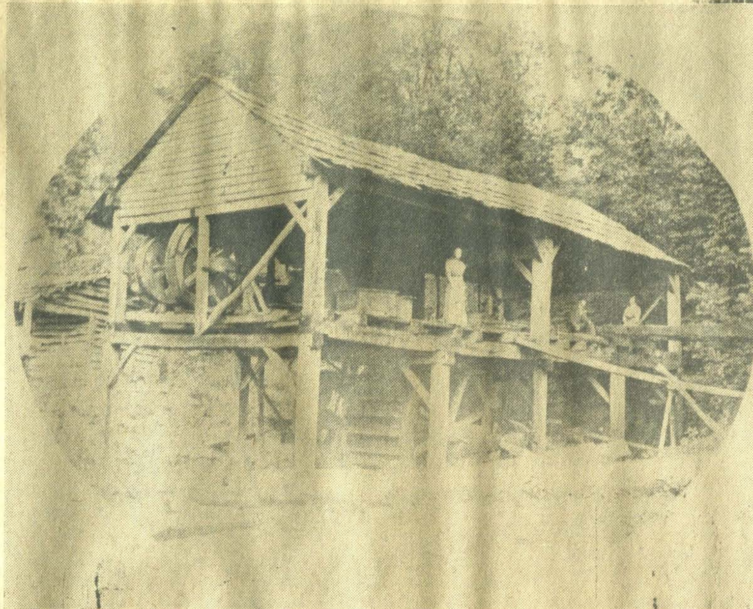
The Leslie grist and saw mill, powered by the diverted waters of Johns Creek in a manner similar to that of the Combs mill at Dwarf on Troublesome Creek, served a wide area for over half a century. This picture was taken in the 1890's.
