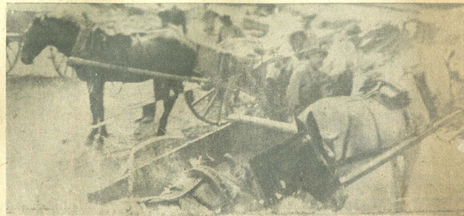
RAILROAD CONSTRUCTION AT COLONIAL
