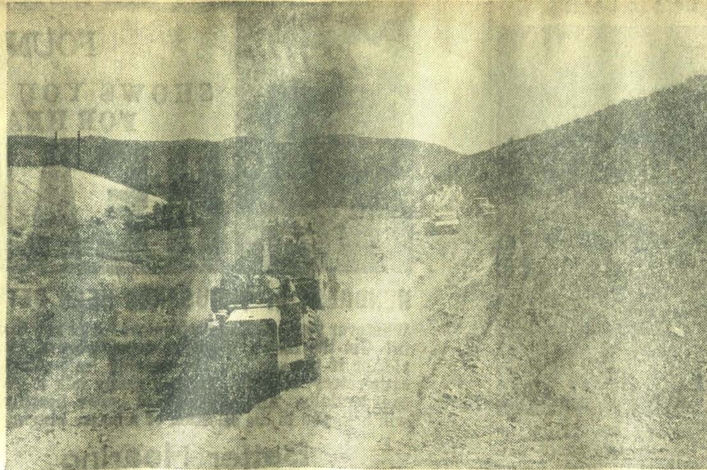
CUT AND FILL is the order of the day on the Eastern Kentucky Turnpike as these heavy construction machines, part of 350 such pieces at work on that project, have moved some 4 million cubic yards of dirt. More than 13 million cubic yards will have been moved when construction is completed December 1, 1962.
