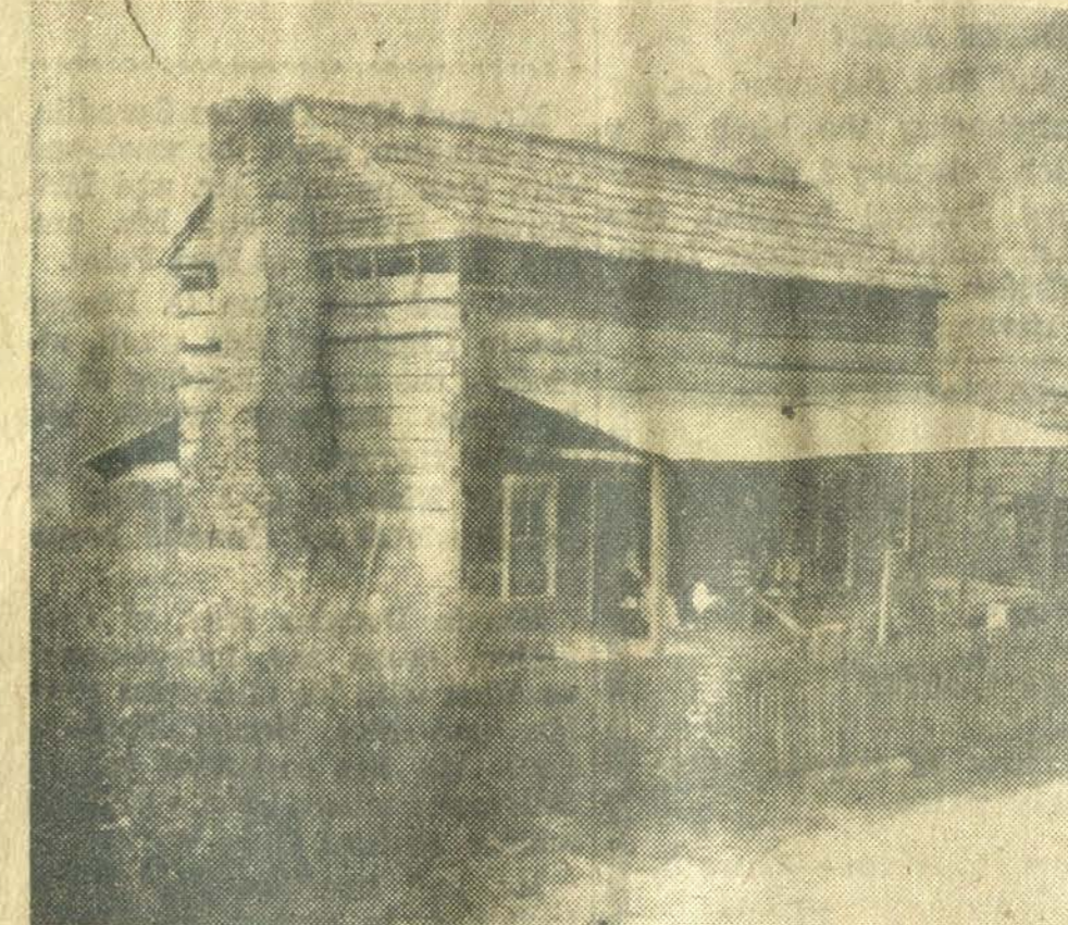
The hewed poplar log, two-story house built by Green Jackson early in the last century on Johns Creek, is typical of thousands of homes erected by well-to-do pioneers of the valleys of the Cumberland, Big Sandy, Licking and Kentucky rivers. The rear lean-to and the front porch here are modern additions. This house, still inhabited, is approximately a century and a half old.
