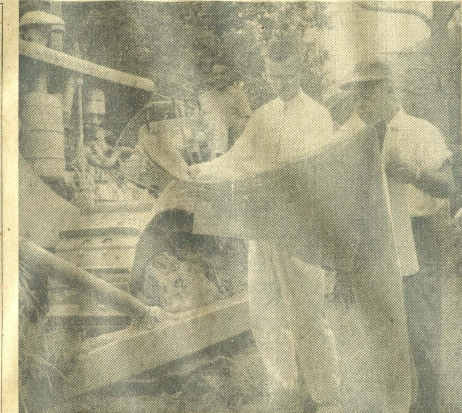
Jack T. Hatcher, Pikeville architect, and Ervin Akers, of Akers & Akers, contractors who will construct the 36-room lodge in Jenny Wiley State Park, go over construction plans as James H. Porter, dozer operator awaits orders to begin moving earth at the lodge site last Friday afternoon.
