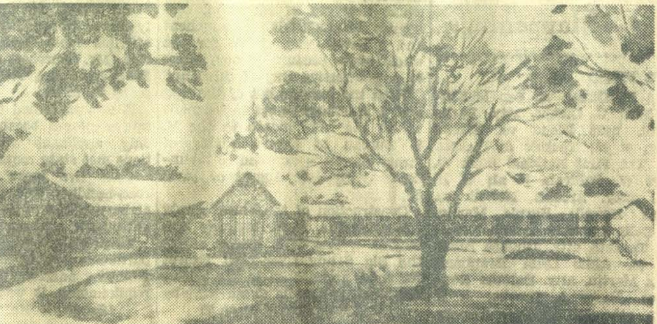
CONSTRUCTION IS UNDER WAY on a 24-room addition (at right) to the lodge at Pennyrite Forest State Park. A new dining room will accommodate 200. The rooms will have terraces overlooking Pennyrite Lake. Native stone exterior will harmonize with the present lodge.
