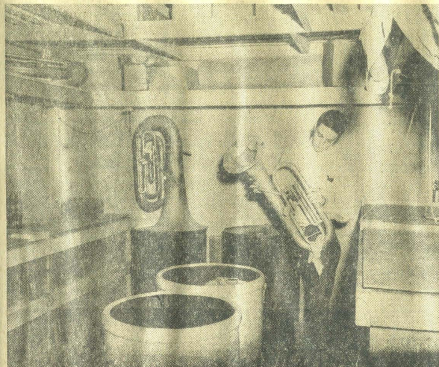
THIS ROOM IS EQUIPPED WITH CROCKS AND LEAD LINED TANKS—For sterilizing, stripping old lacquer and brightening brass and silver, corrosion removed from slides.
