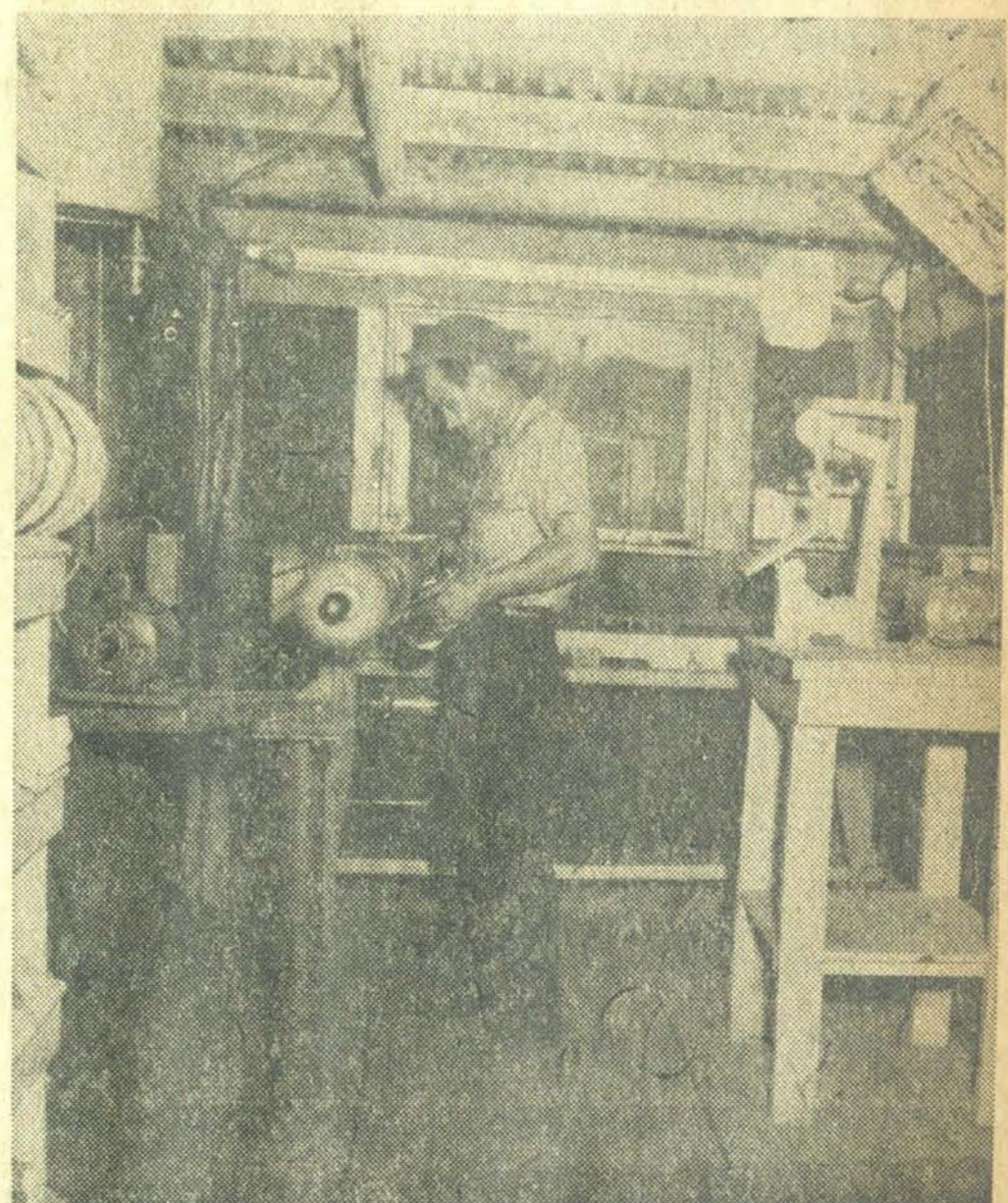
THIS IS THE BUFFING AND SCRATCH BRUSHING ROOM And where broken barrels and tenor joints of clarinets are built. When brass or silver, done in this department, they have been brought to a high luster sheen.
