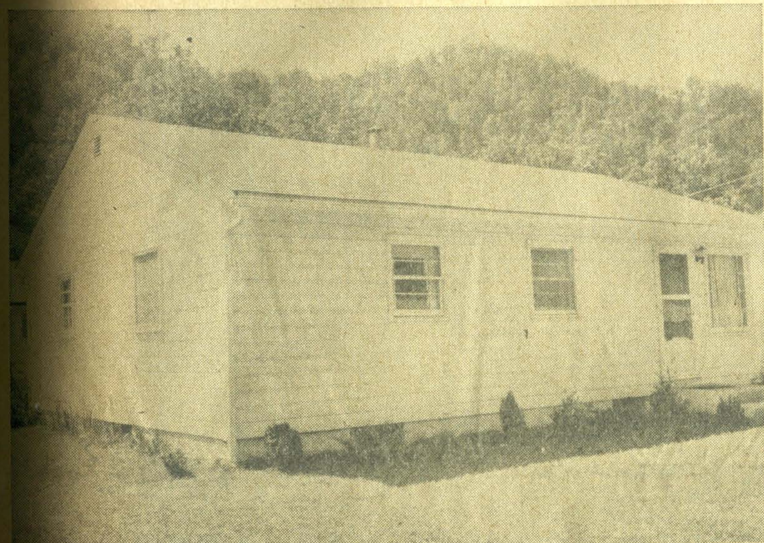
Full Basement (finished) — Three Bedroom — Wall-to-wall Carpeting — Built-in Kitchen, complete with Oven and Range — Paved Driveway — Complete with shrubs and lawn
