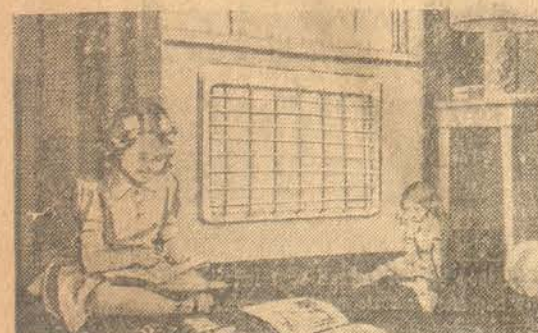
WALL TYPES. Panel type heaters radiate heat rays. Convection and fan type heaters circulate warmed air. Use them for heating a single room or an entire house. All come in portable or wall-mounted styles.
