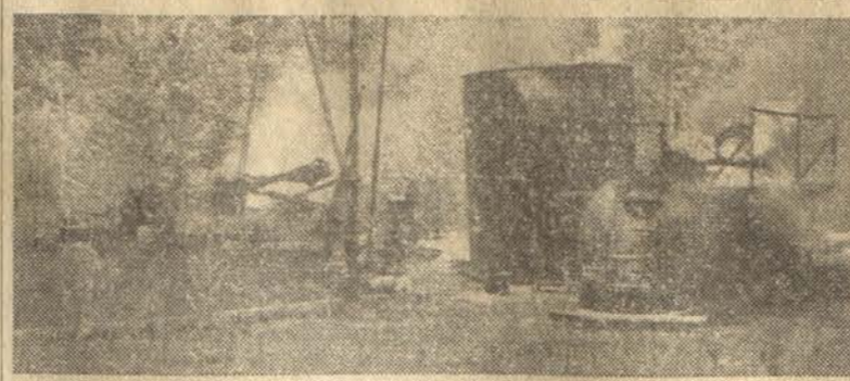
This was the scene at oil well fire: At left, truck-mounted drilling rig; center, oil well pump; right center, 100-barrel oil storage tank. At right is 2,000-gallon sand-and-oil-mixing tank, belonging to Dowell, Inc., oil well service company. Picture was taken about two hours after the fire started.
