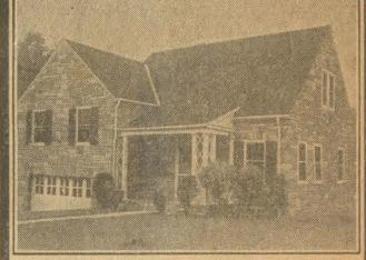
· PERMA-STONE encases the building from the ground u in a stone-like, weather-proof, steel reinforced, concrete armor, which greatly strengthens the walls.
