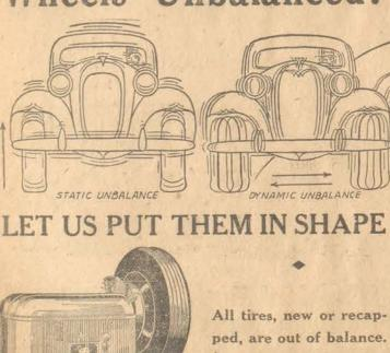
ped, are out of balance. By balancing, tire mileage is increased and wear and tear on your car is decreased.
